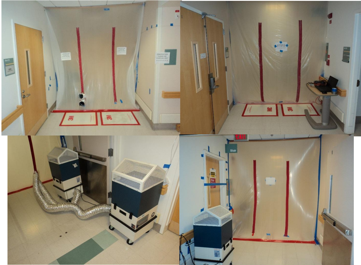
Figure S1. Pictures of the temporary anteroom installment: (top left) external ingress view, (top right) external egress view, (bottom left) internal ingress view, and (bottom right) internal egress view.
